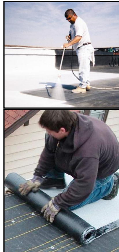
Figure 6: Two Cool Roof Installations
