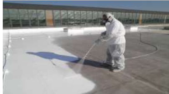
Application of Cool Barrier Reflective Coat using an airless spray
