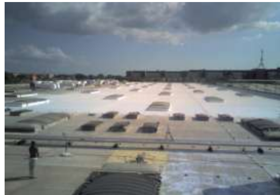
Application of Cool Barrier Reflective Coat using an airless spray
